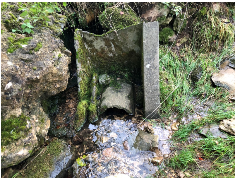
Site 4 – Pipe culvert
