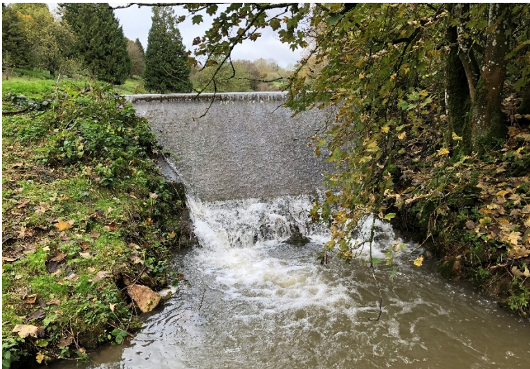
Site 6 – Large, man-made concrete weir with a vertical drop.
