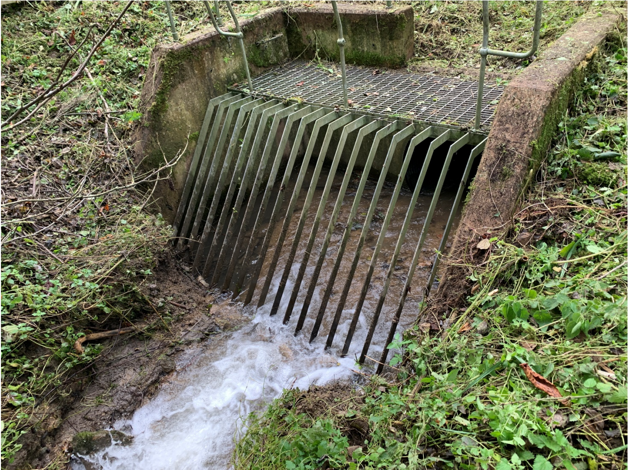
Figure 3-3 Existing culvert entrance under A417 - Tributary of Norman's Brook
